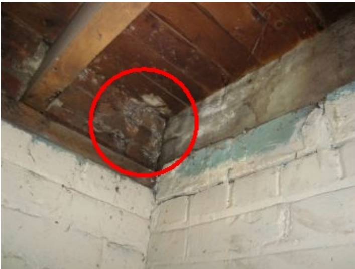
Efflorescence
